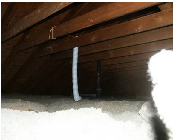
Bathroom exhaust - venting into attic
