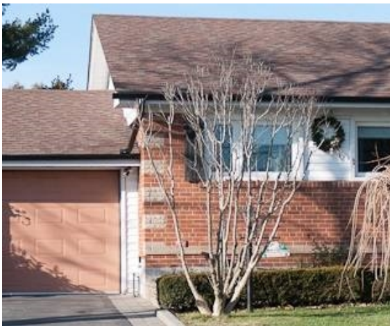
Shows upper gutter draining into lower gutter
