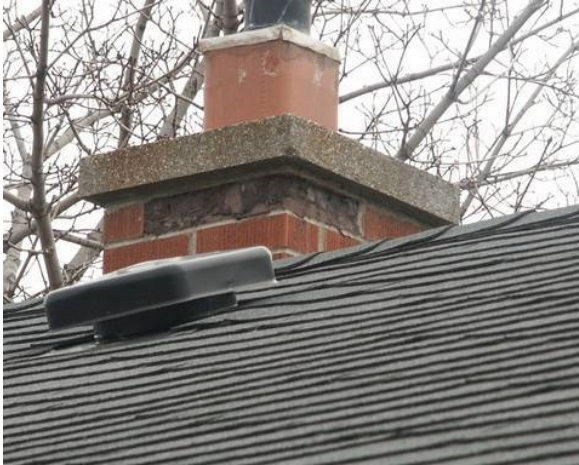
Minor brick damage
