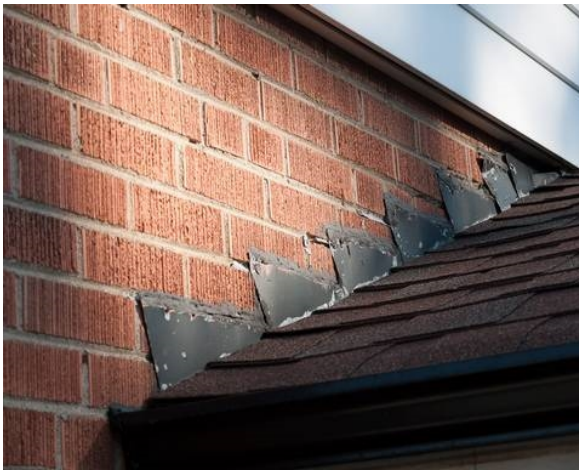
Roof to sidewall flashing
