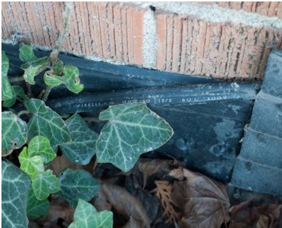
Exposed electrical cable at east side of home in garden
