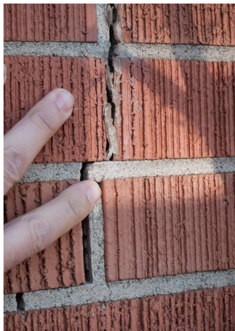
Settlement crack at west wall of garage
